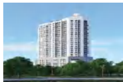
HR1 BUILDING Product name: SIVACON S8
